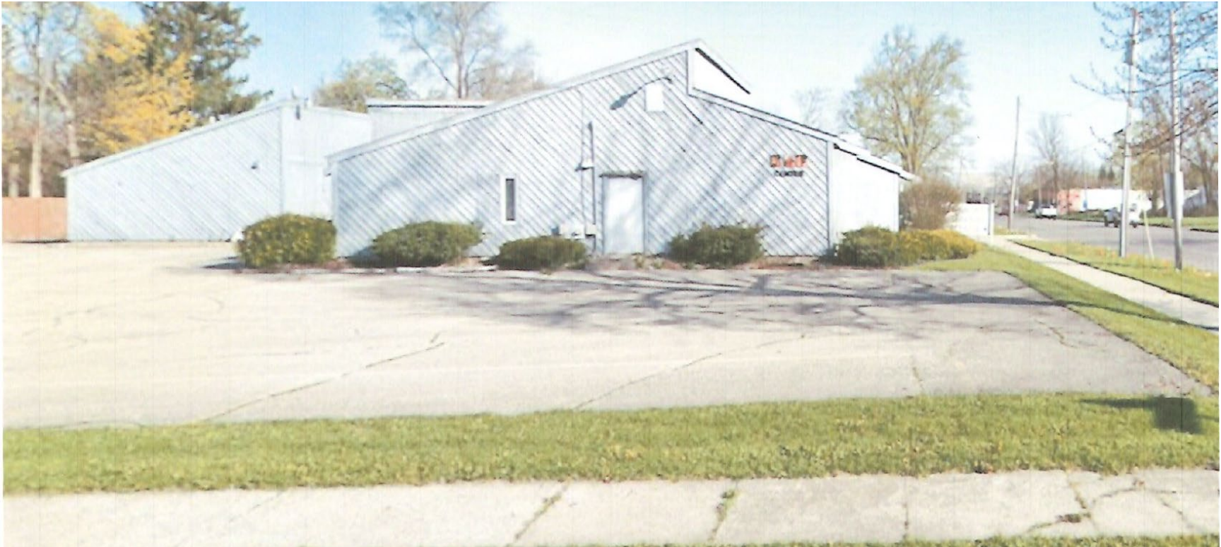
South side: Facing building
