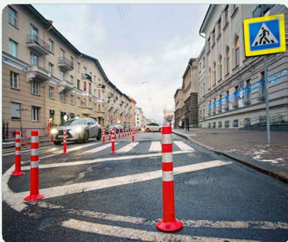
Transverse Striping and Flex-Post/Bollard Curb Extensions Photo courtesy of Tricky Shark/Adobe Stock
