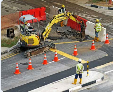
Intersection Realignment Photo courtesy of Ceogh/Freerange Stock
