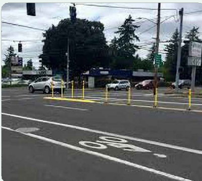
Hardened Centerline Photo courtesy of Portland Bureau of Transportation/ Creative Commons
