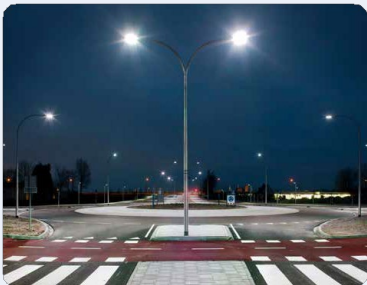
Intersection Lighting/Illumination Photo courtesy of Peter de Kievith/Adobe Stock
