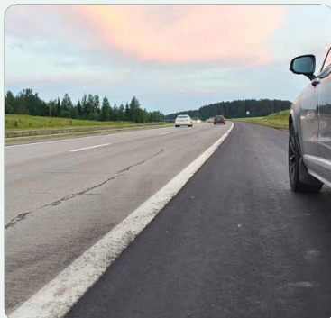
Paved Shoulder Photo courtesy of Balsem/Adobe Stock
