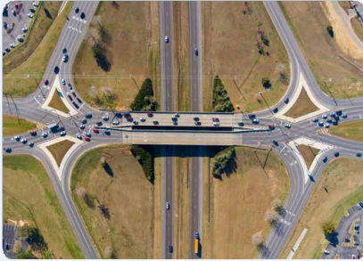
Diverging Diamond Interchange (DDI) Photo courtesy of George/Adobe Stock
