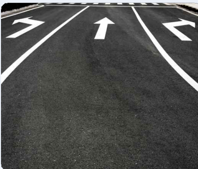
Dedicated Left and Right Turn at Intersections
