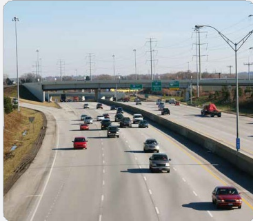
Median Barriers Photo courtesy of Kenneth Sponsler/Adobe Stock
