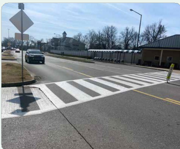
Crosswalk Visibility Enhancements
