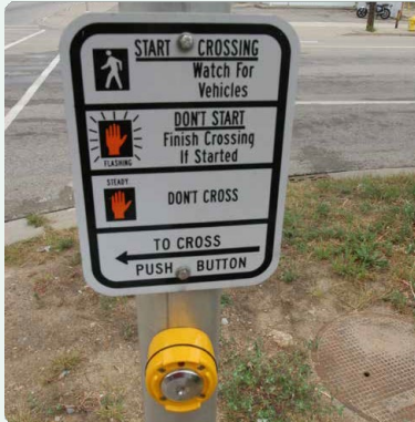
A pedestrian push button allows pedestrians to activate a pedestrian signal and reassure pedestrians that they will receive a crossing indication. Source: pedbikeimages.org - Dan Burden (2006)
