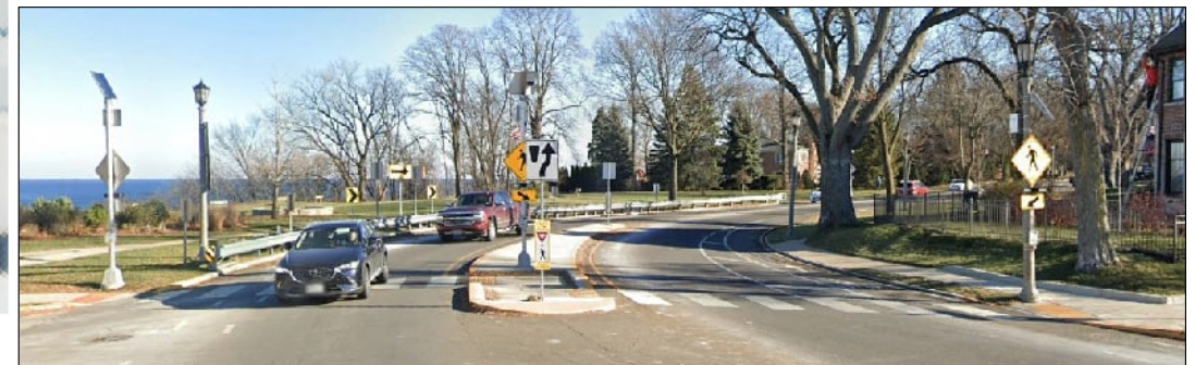
MID-BLOCK PEDESTRIAN CROSSING WITH STAGGERED MEDIAN AND RRFB PEDESTRIAN PUSHBUTTONS
