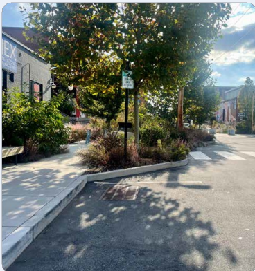
Concrete Curb Extension Original photo taken in field
