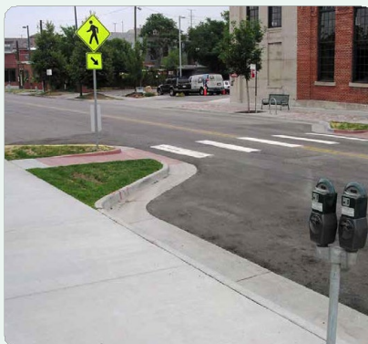
Intersection/Mid-block Curb Extension/Bulb-out Photo courtesy of Richard Drdul/Wikimedia Commons
