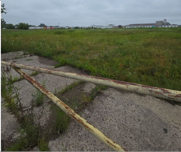
Subject property, south side of subject property
